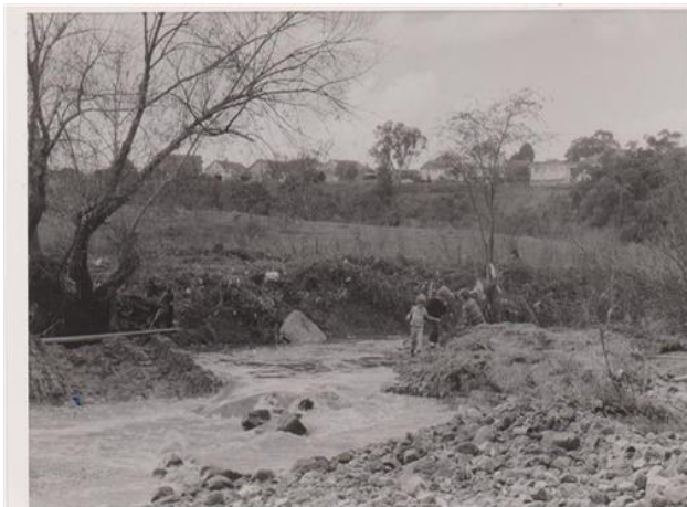
Photo showing the initial works of Clifton Bridge -1974
