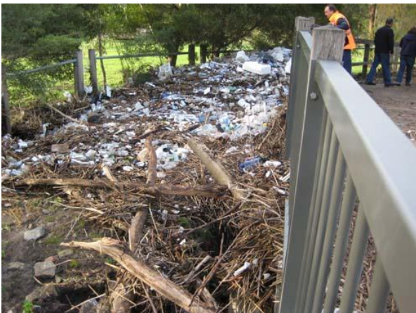
Daunting rubbish pile at Willowbank Bridge
